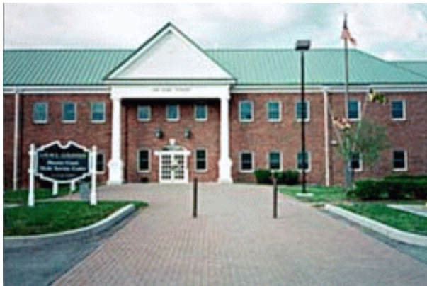
Calvert County District Court
